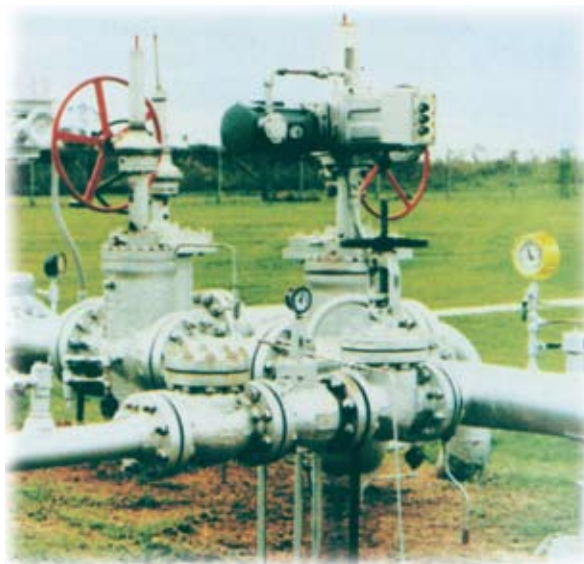
M&J Valve surge relief system protects pipelines from transient pressure surges
